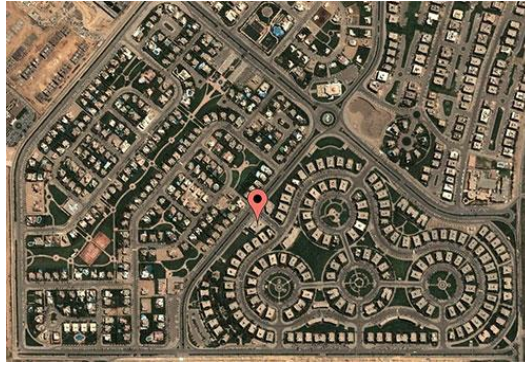
Fig. 16. Beverly Hills compound, El-sheikh Zayed [32]
