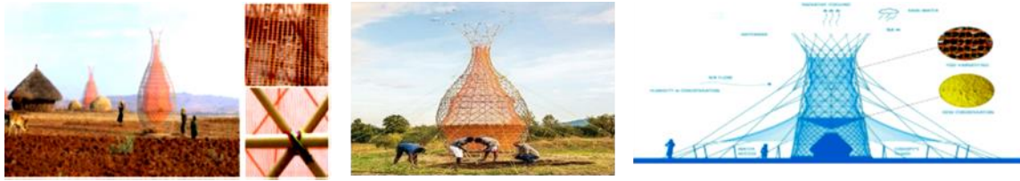
Fig.15 Implementation of Water Management Strategies Inspired by Spider, Cactus Thistle and Namib Beetle in Project Warka Tower [38]
